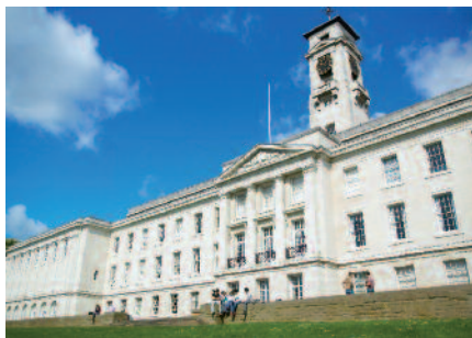
Trent Building, University Park
