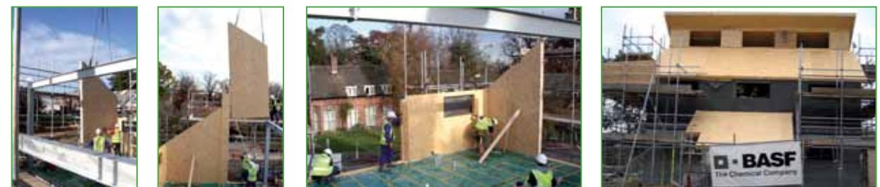
A prefabricated timber insulated sandwich panel containing rigid polyurethane foam insulation has been used on the house. This material has been chosen because of its lightweight, high insulation factor and the ability to prefabricate off-site non-rectangular shapes i.e. to the gable walls. The roof is constructed of the same material. This avoids the need for a separate roof structure, as one would need for a traditional build.
