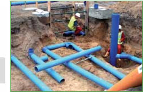
REHAU has developed the first ground to air heat exchanger with an antimicrobial inner layer which, as well as saving both costs and energy, will ensure a considerable improvement to the quality of air.
