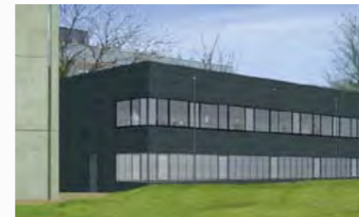
A new £1.5m Aerospace Research Centre extension to the existing Tower Workshop will incorporate workshop and office spaces. To be completed by September 2010.
