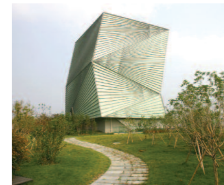
CSET building in China
