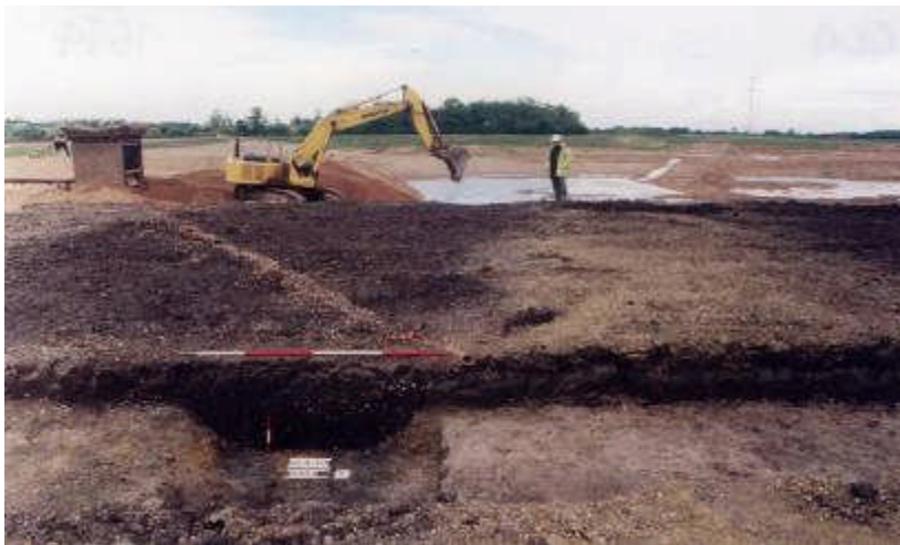
Valley landscapes: Gonalston, Nottinghamshire. Iron Age boundary ditch flanked by sub-alluvial gravel bank. Photograph: L. Elliott
