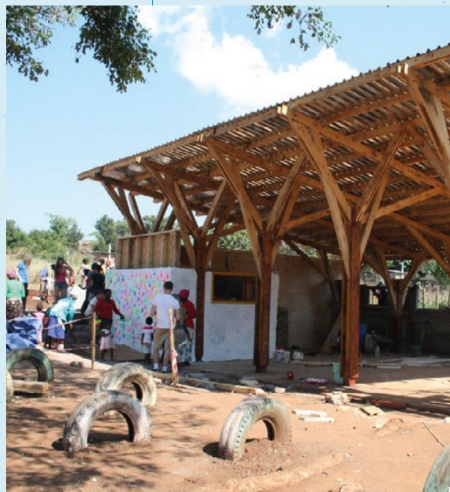
Khomotso Crèche phase 2 (2013), 4 classrooms and 124 children.
