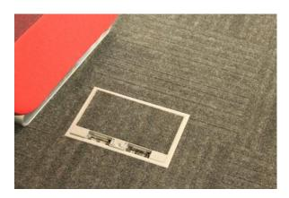
A further item related to the floor boxes in the Graduate Centre to house the electrical sockets. The retractable hoods shielding the cables are easily broken causing potential trips and a hazard to those wearing narrow heeled shoes. The use of this type of floor box should be avoided and alternative cable management methods considered.
