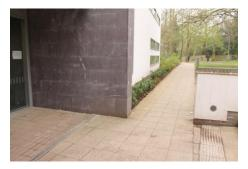
Users have experienced flooding of the lobby area in heavy downpours of rain due to blockage of the drainage channel. A larger channel section together with an additional drainage channel across the adjacent path would have been a better solution.
