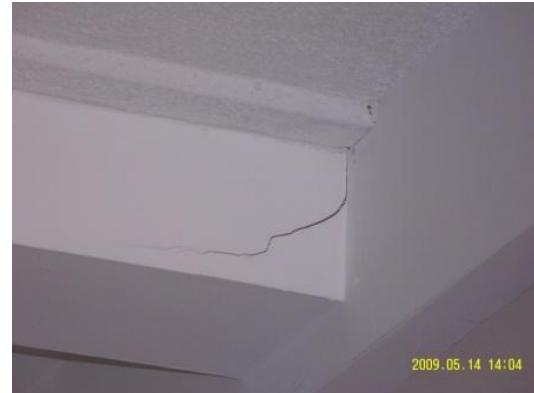
There was evidence of cracking due to some settlement/shrinkage shortly after handover of the building. Remedial work was carried out including redecoration. It was observed during a recent tour of the building that movement is still occurring with evidence of cracks in masonry and plaster in a number of areas.
