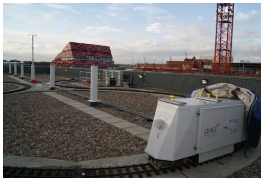
Test Track area on roof
