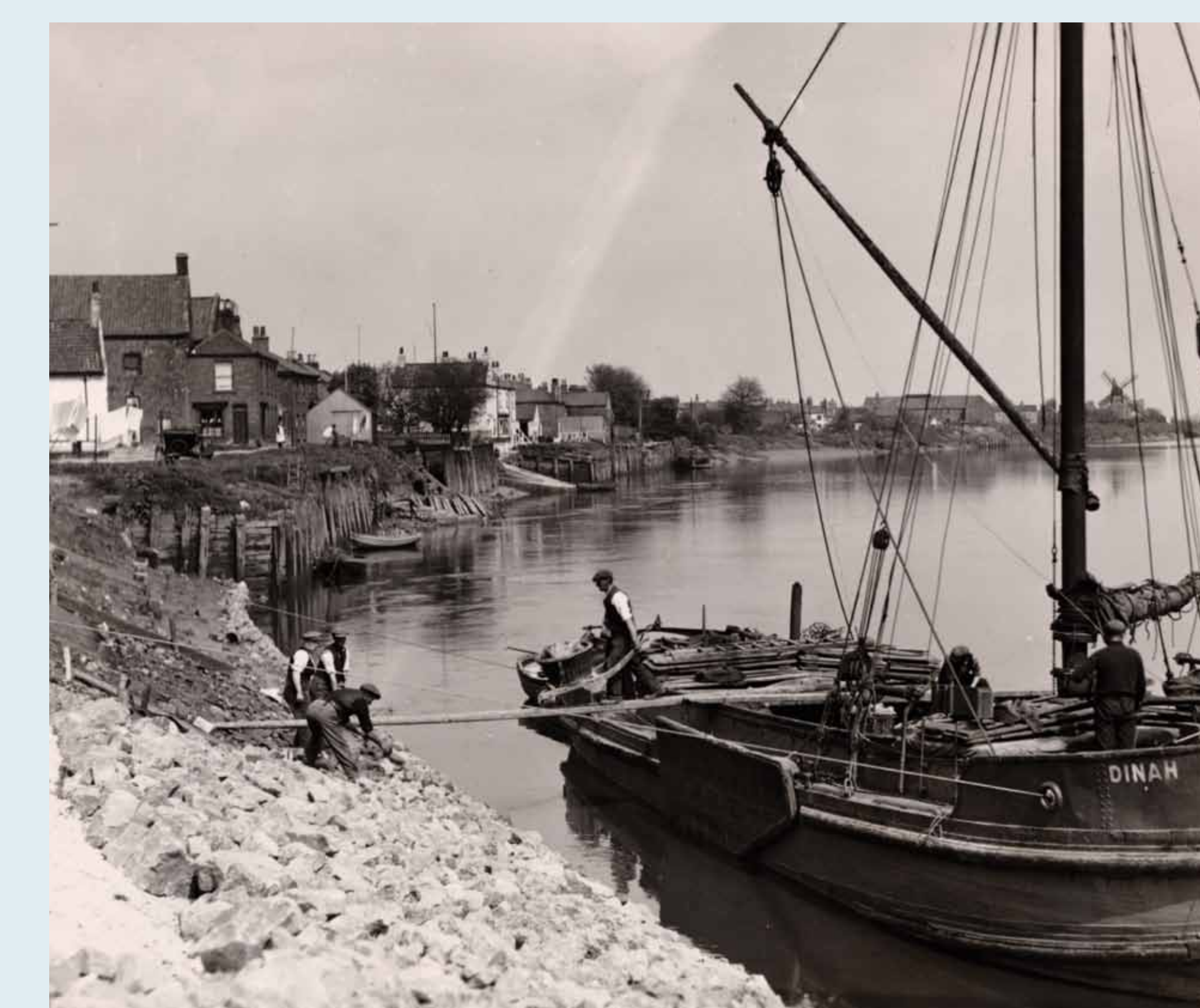
Revetting work at Owston Ferry, 1935 Records of the Trent River Authority, RE/DOP/X/1, p.62
