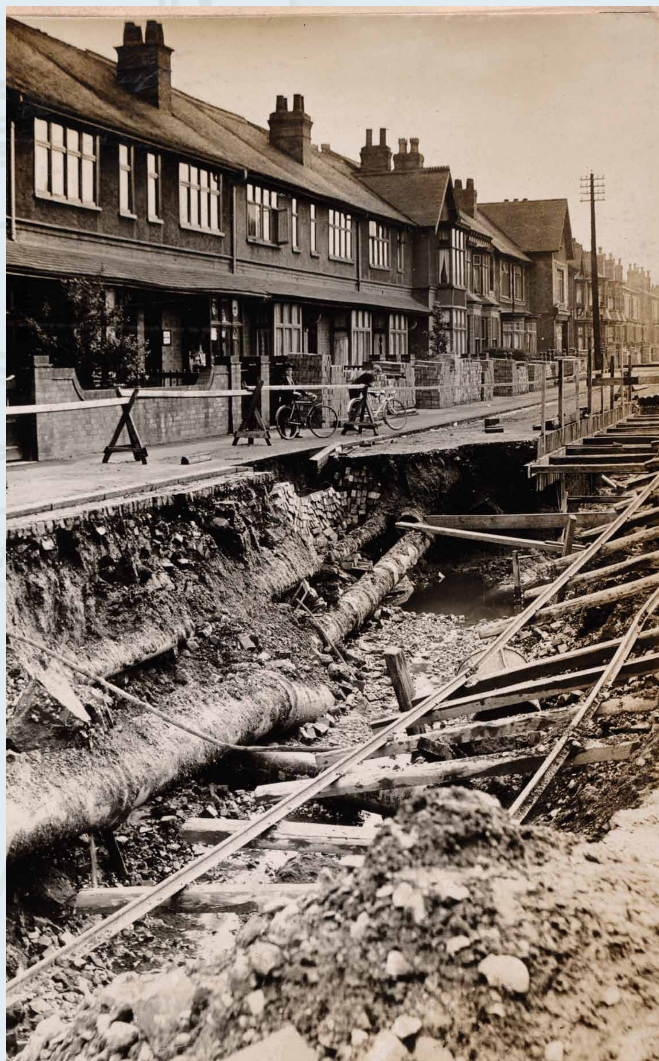
Photograph of burst 12 and 18 inch water mains at Haydn Road, Nottingham, 1914 Records of the City of Nottingham Water Department, R/HR/1/8/1/164
