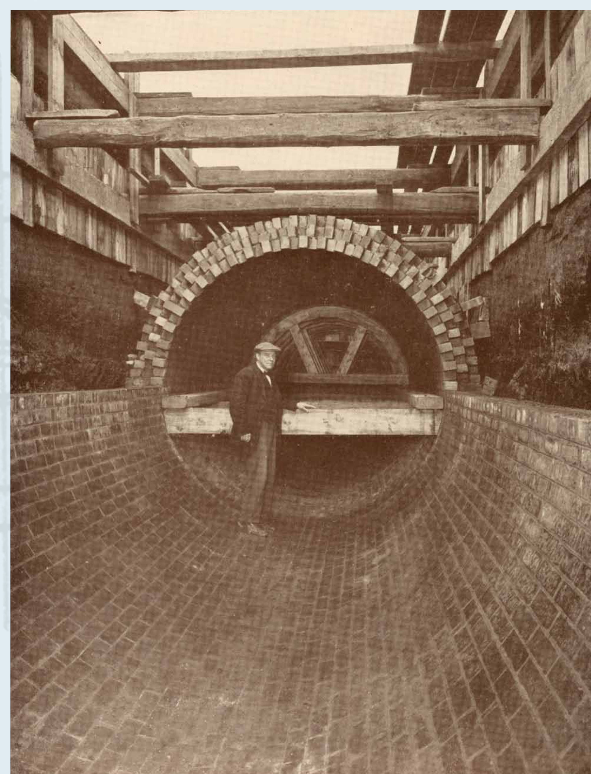
Construction of new main sewer at Bobbers Mill, Nottingham, 1936 East Midlands Collection o/s pamphlet Not 3.G66 NOT
