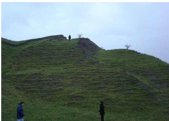
Figure 3.5. Landslide of the Miege spoil - Pechelbronn mine, France (Image courtesy of Ineris)
