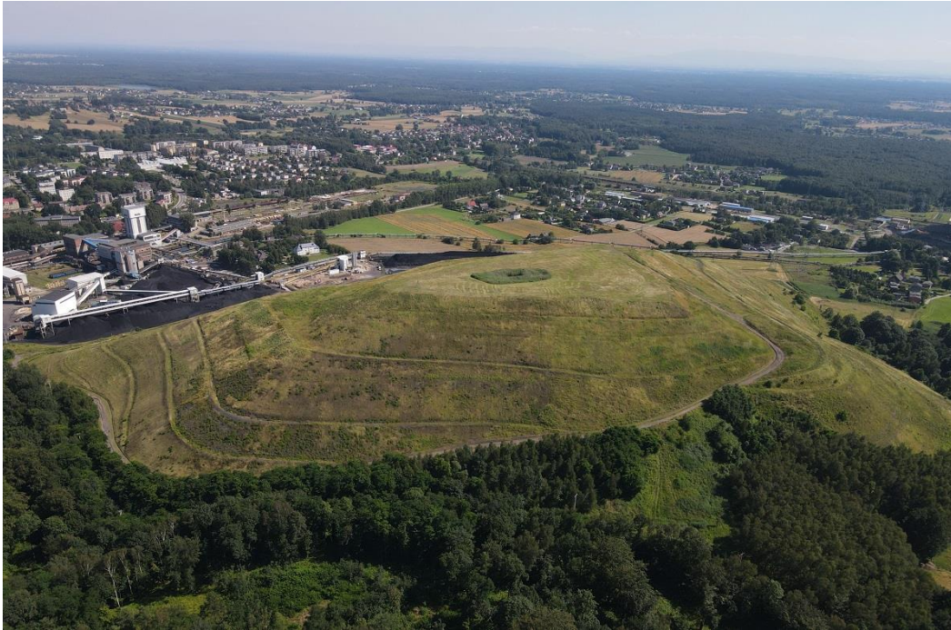
Figure 3.4. The "Skalny" spoil located next to the hard coal mine in Łaziska Górne, S Poland - one of the largest spoils in Europe with a volume of 15.5 million m 3 and a height of 92 m (Image courtesy of GIG).
