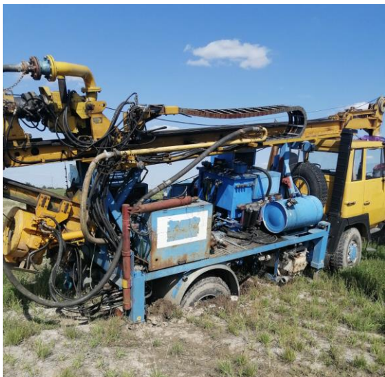
Figure 5.2. View of a testing machine becomes stuck in the soft spoil material.
