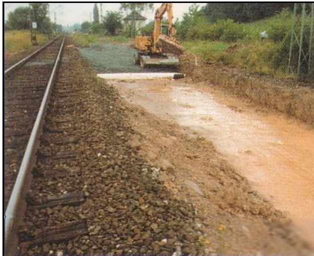
Figure 2.30 Installation of polymer grid (Tensar International, 2001b)
