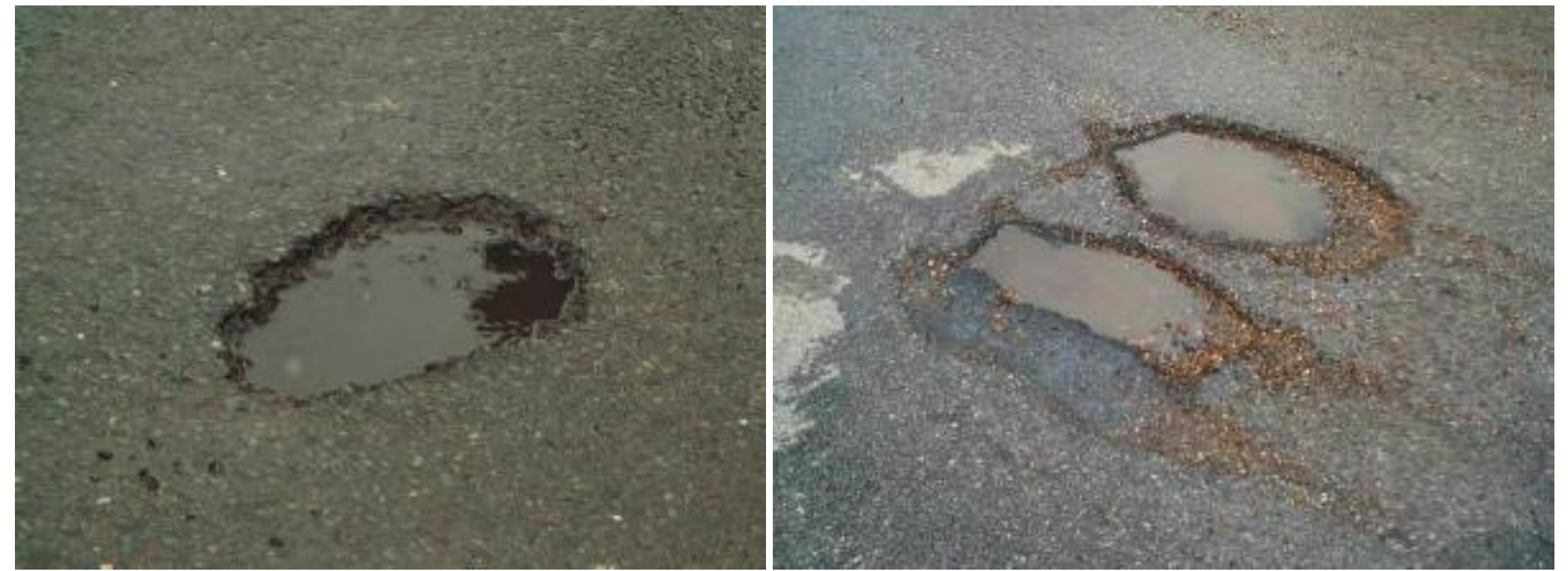
Figure 1: Fracture Pothole and Attrition Pothole
