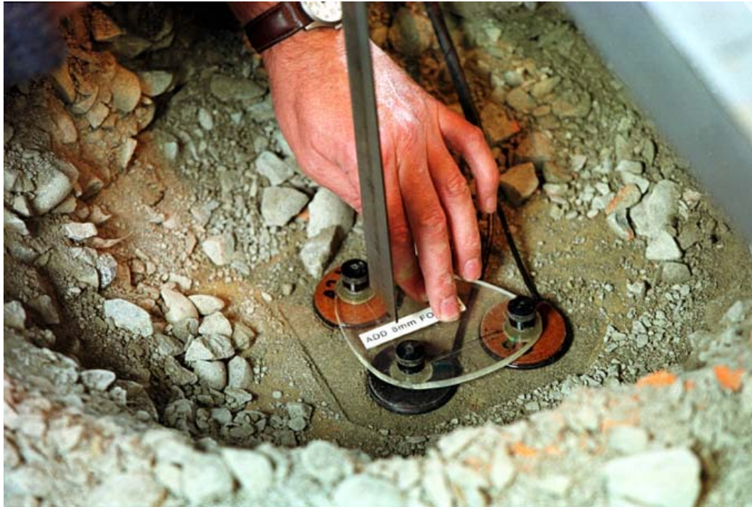
Figure 4.8. Emu strain coil installation.
