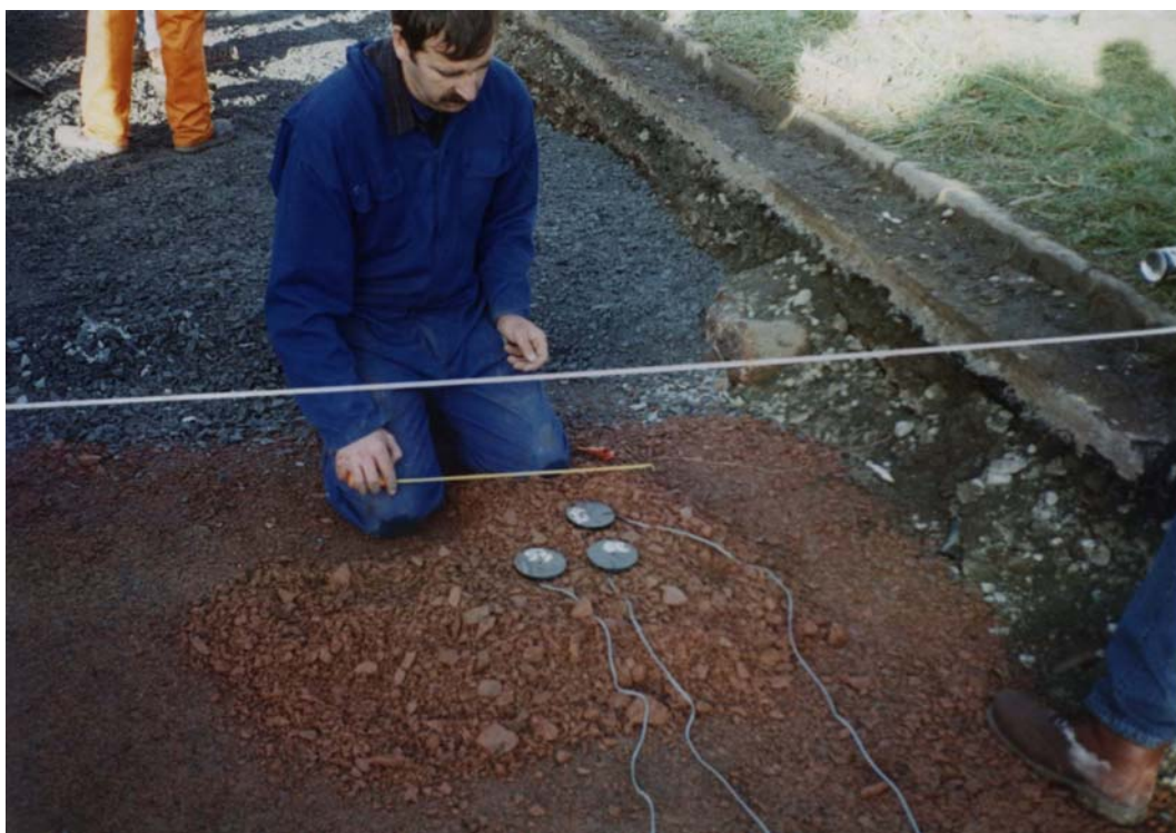
Figure 5.11. Emu strain coil installation.
