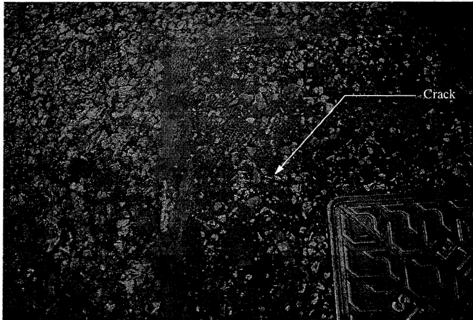
Figure 3.8: Deterioration of the HRA surrounding the north manhole
