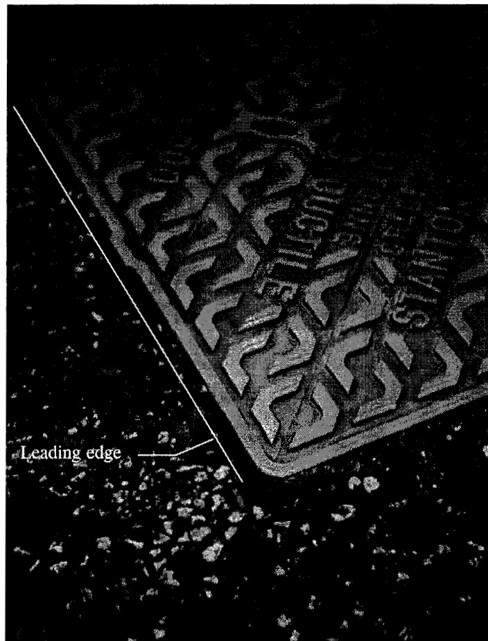
Figure 3.5: Deterioration of the HRA along the leading edge
