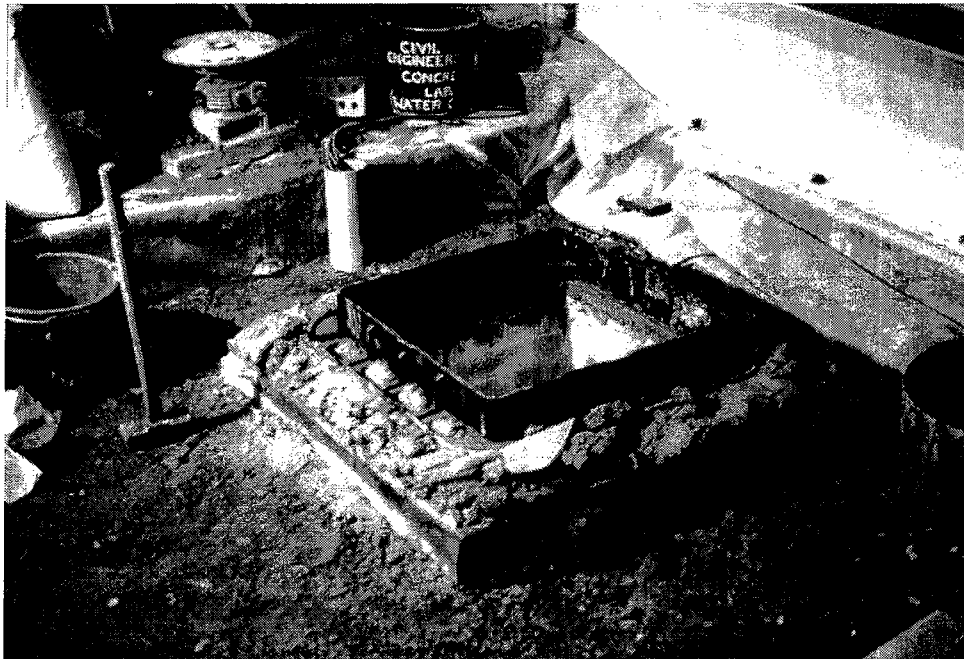
Figure C.8: Installation of bedding layer on top of quarry tiles and frame prior to tamping
