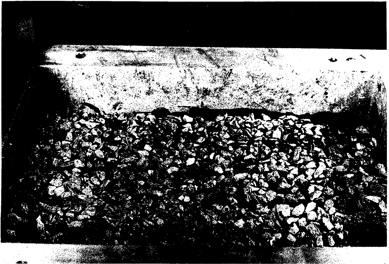
Plate 3.2 (a) Completed Interlayer Treatment for the Geogrid
