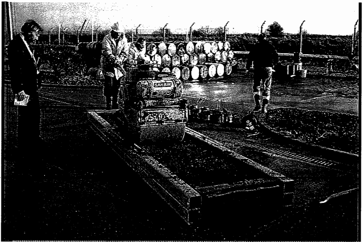
Figure 7.17 Compaction of Slab
