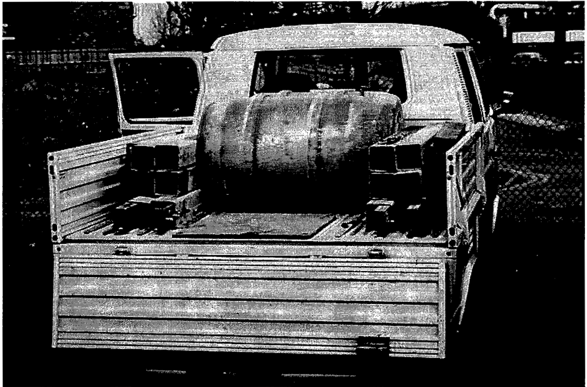
Figure 7.2 Formwork Dismantled for Transportation
