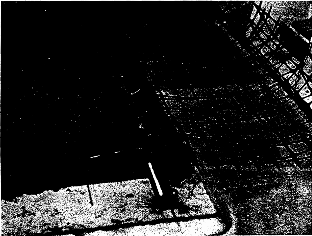
Fig. 7.3 Grid anchored with a reinforcing bar
