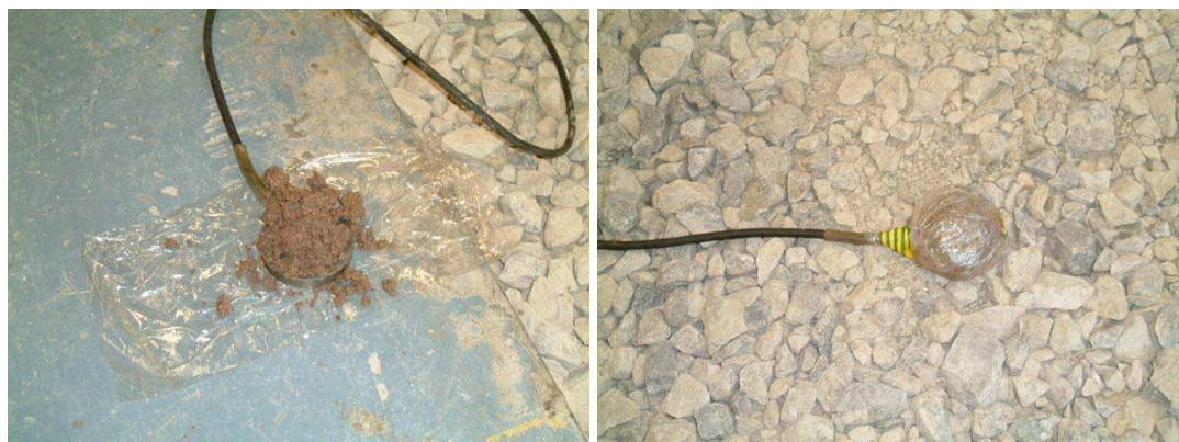
Figure 6.9 Installation of a pressure cell
