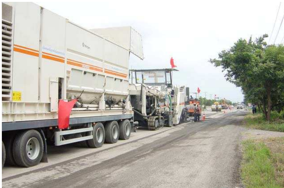
Figure 1.3 A recycler and a slurry mixer in operation.
