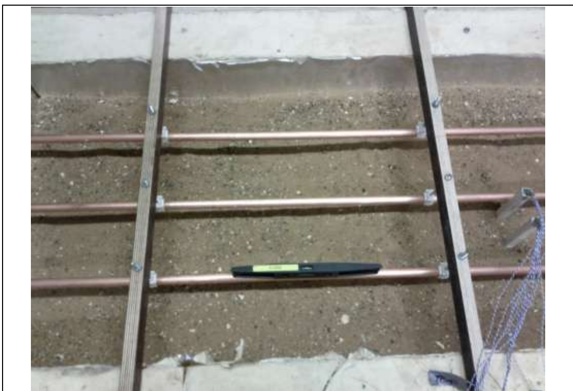
Figure 5-7 Supporting and levelling the collector pipes
