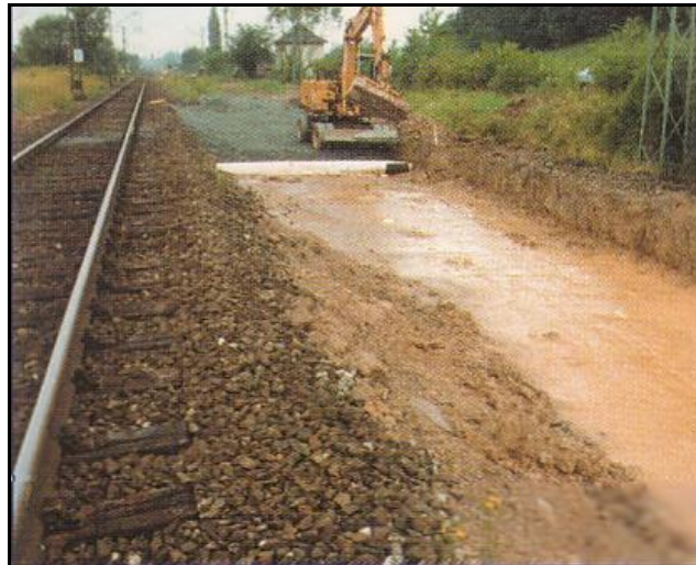
Figure 2.30 Installation of polymer grid (Tensar International, 2001b)
