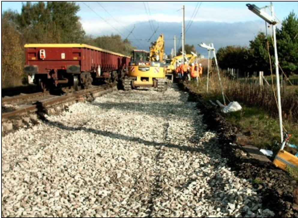
Figure 6.1 Renewal work at Coppul Moor
