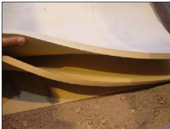
Figure 4.3 Very soft subgrade conditions in CET
