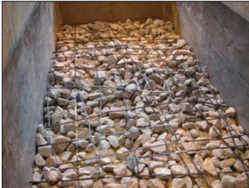
Figure 4.29 Broken grid junctions
