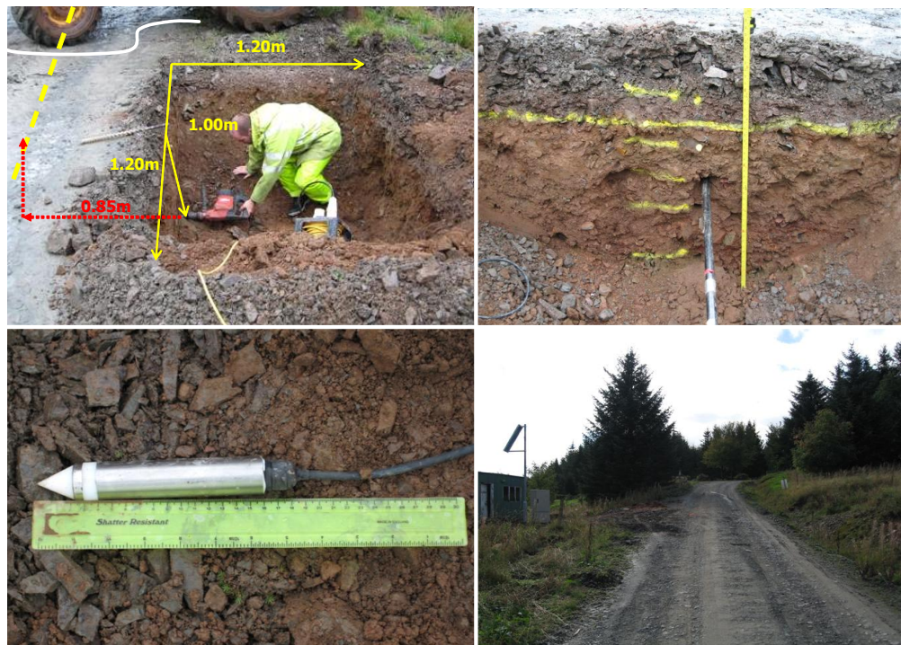
Figure 4.37 – Percostation installation at Till Hill Main Block entrance – off B709 Eskdalemuir/Scotland
