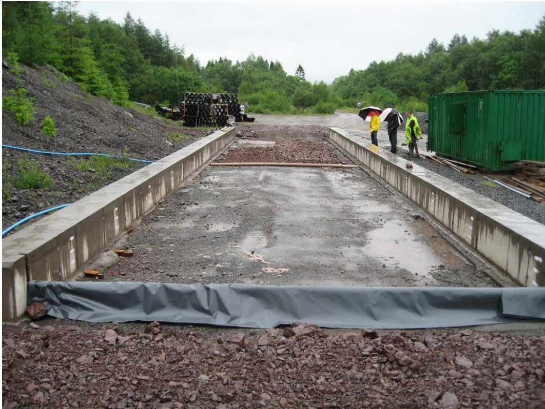
Figure 4.14 – Barrier at both ends of the walls to contain water
