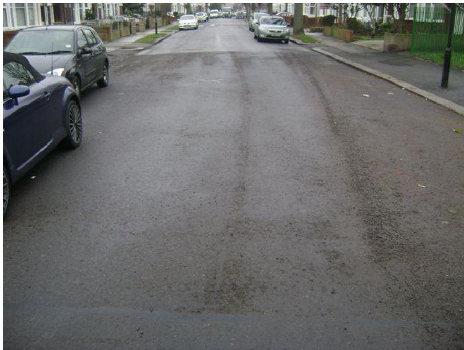
Figure 7.28 – Photograph showing the onset of fretting particularly in the wheeltracks
