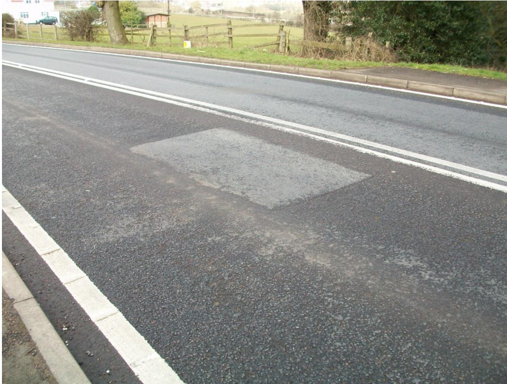
Figure 7.13 – Photograph of patch repair and onset of minor fretting (March 2010) on anti-icing surface (bottom lane) and control surface (top lane)
