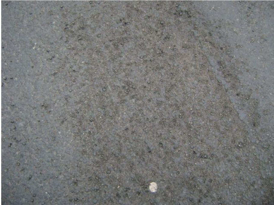
Figure 7.30 – Photograph of minor fretting located in areas where traffic is turning.
