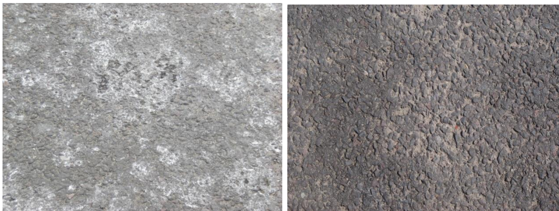
Figure 7.8 - Chemical deposits on surface 15/06/09 (left) and surface after a rainfall event 19/06/09 (right)
