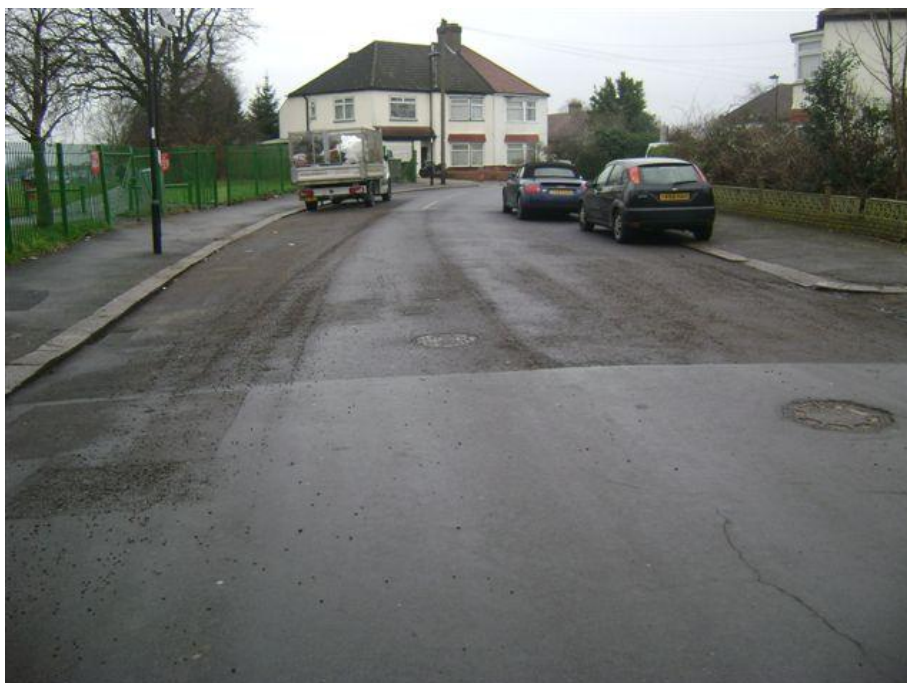
Figure 7.29 – Photograph showing the onset of fretting distribution over the lane width
