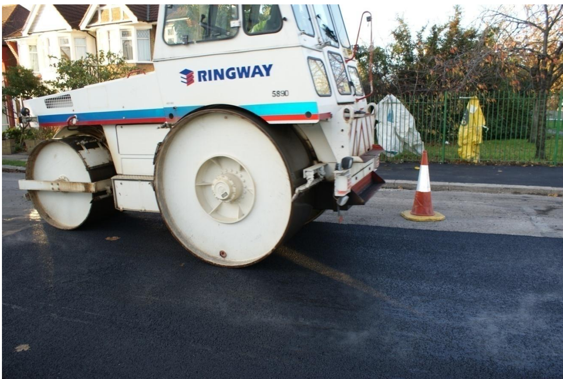
Figure 7.16 – Compaction of anti-icing surface course
