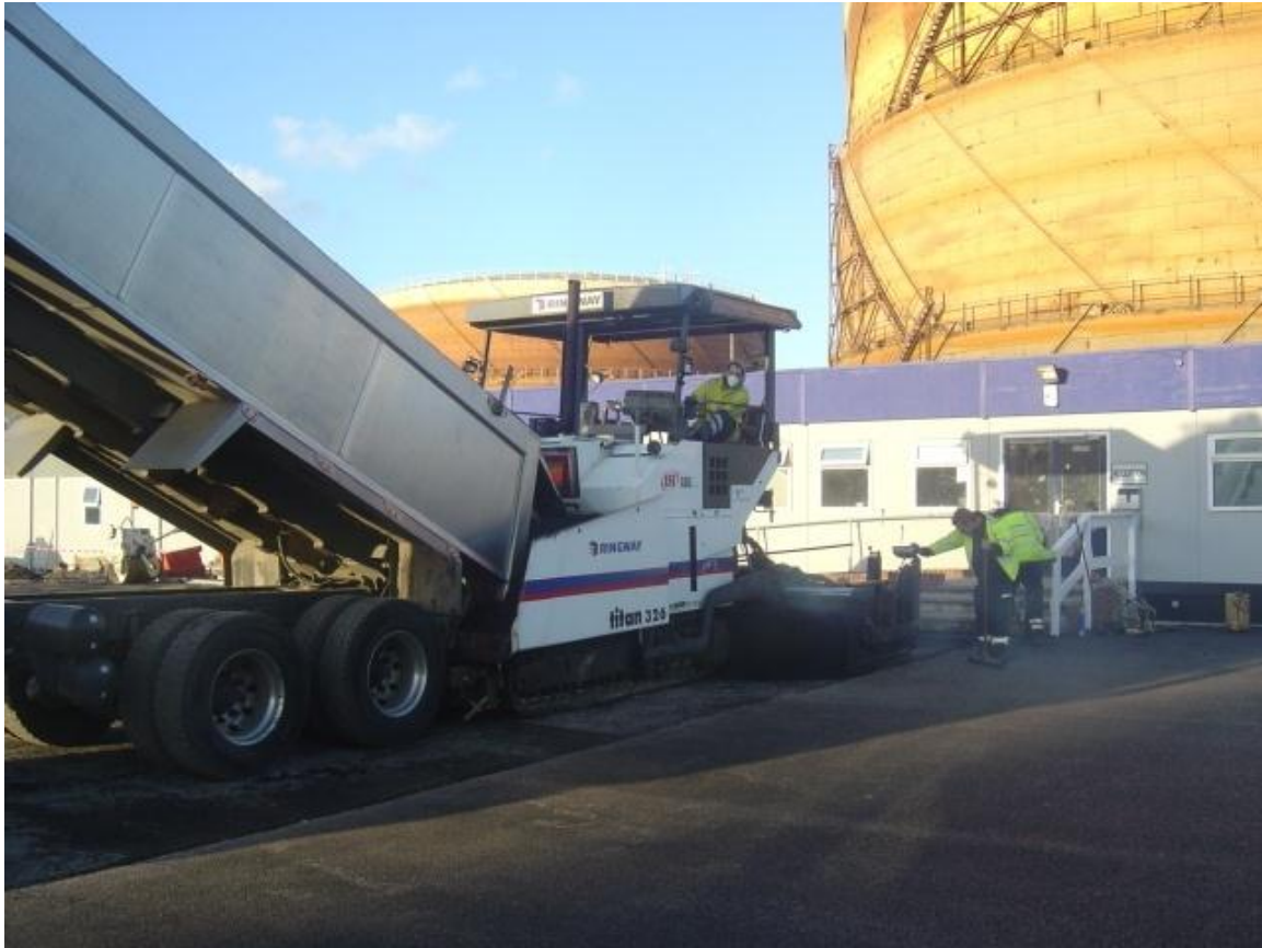
Figure 7.4 – Laying and compaction of anti-icing surface course material
