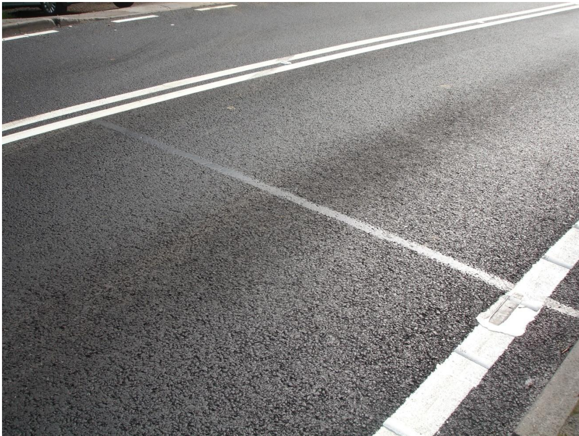
Figure 7.12 – Photograph of the Ridgeway site with the control surface (left lane) and modified surface (right lane)
