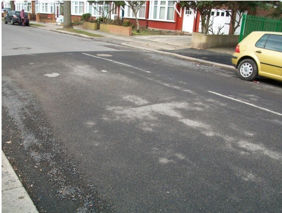
Figure 7.21 – Photograph showing the widespread fretting of the anti-icing surface course
