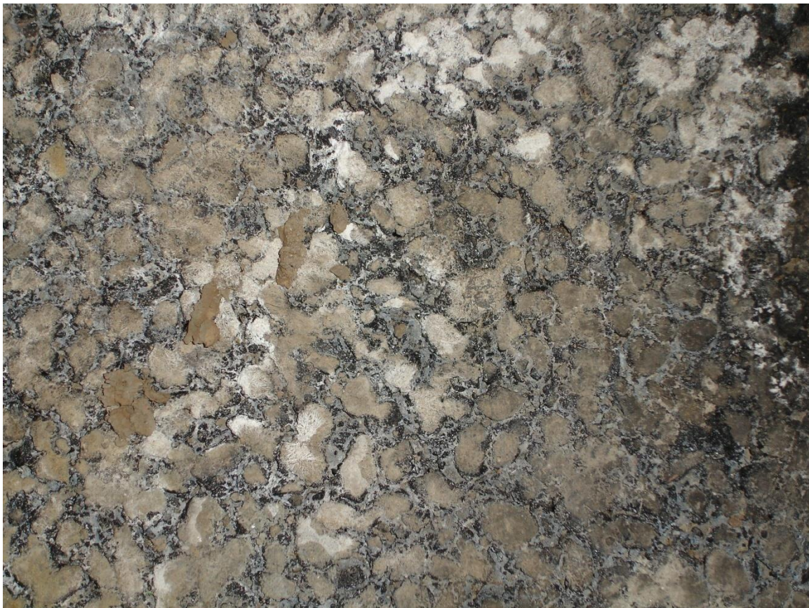
Figure 7.7 – Chemical deposits on surface during low humidity
