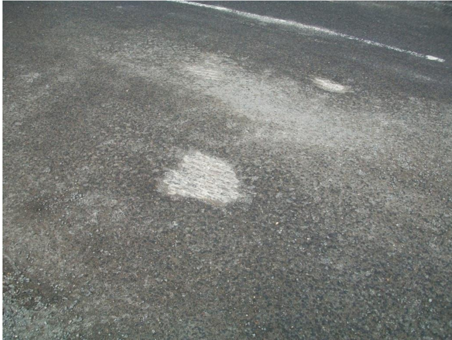
Figure 7.22 – Photograph showing the localised disintegration of the anti-icing surface course through to the underlying base
