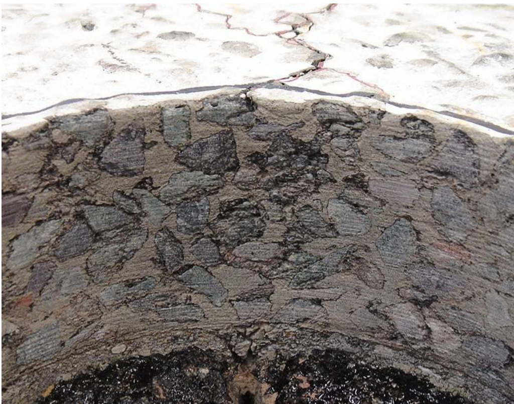
Figure 7.30 – Hole in PTF as a result of extracting a core from the surface course
