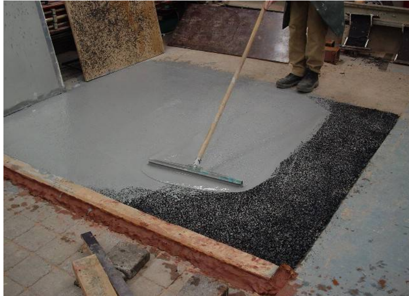
Figure 7.14 – Application of the grout on the first two contiguous sections
