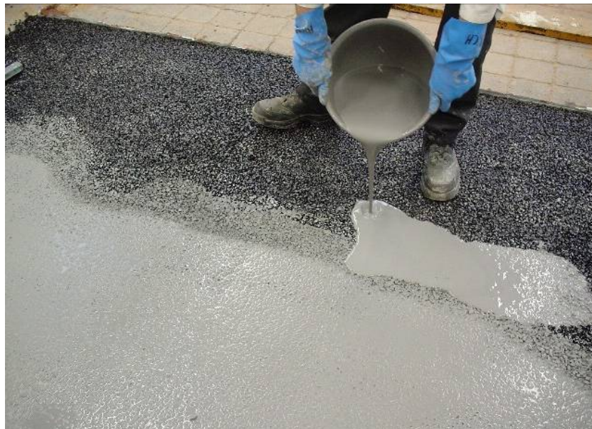
Figure 7.15 – Application of the grout on the third and fourth sections
