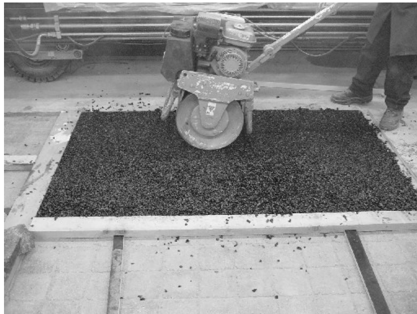
Figure 7.12 – Compaction of porous asphalt in the first section
