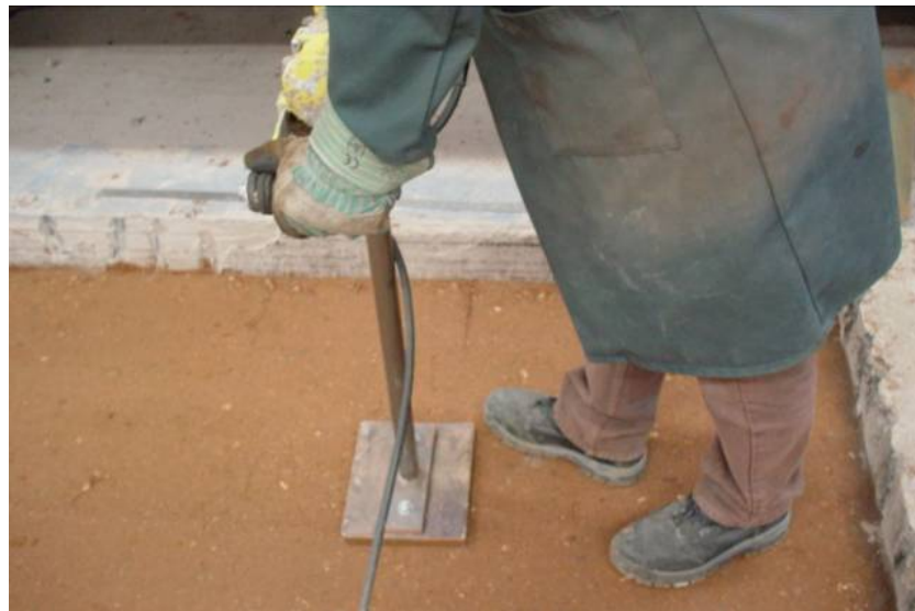
Figure 7.5 – Compaction of PTF granular material
