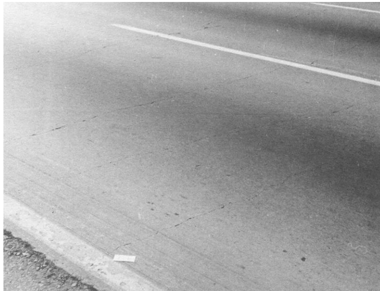
Figure 2.7 – Typical cracking in continuously reinforced concrete pavement (Croney and Croney, 1991)
