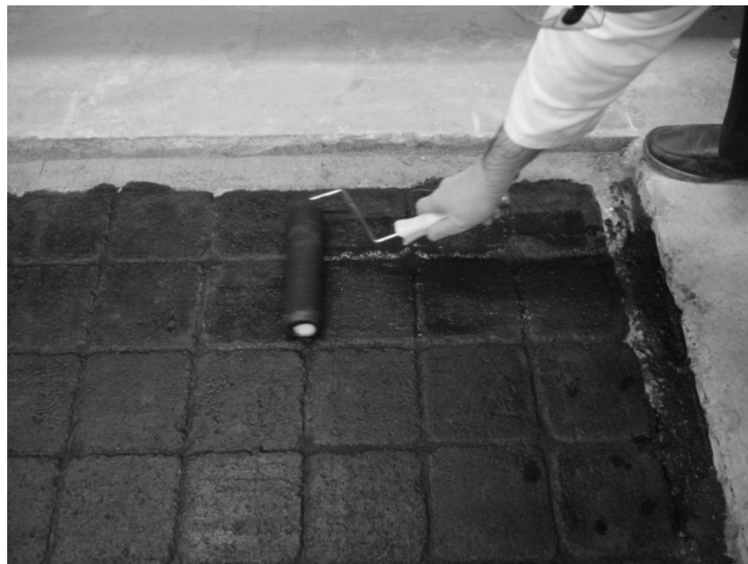
Figure 7.11 – Tack coat application in the first section
