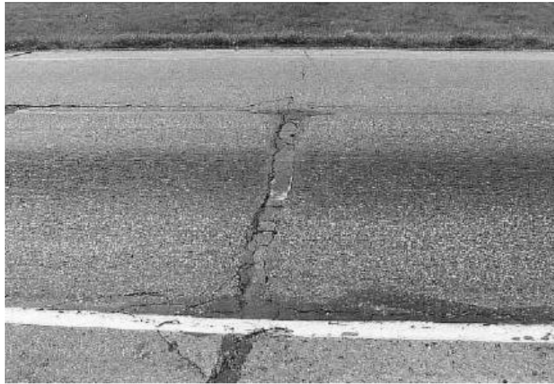
Figure 2.10 – Reflective cracking in a composite pavement with a jointed concrete base (Saraf, 1998)
