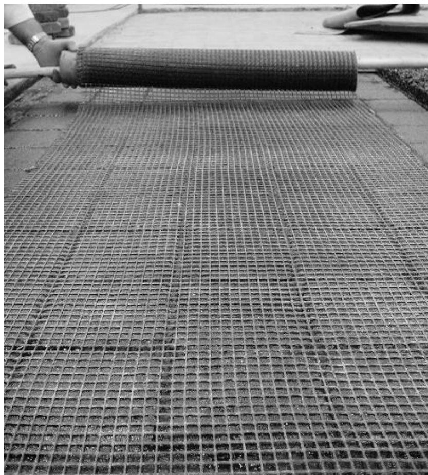
Figure 7.13 – Application of Glasgrid® reinforcement in the second section
