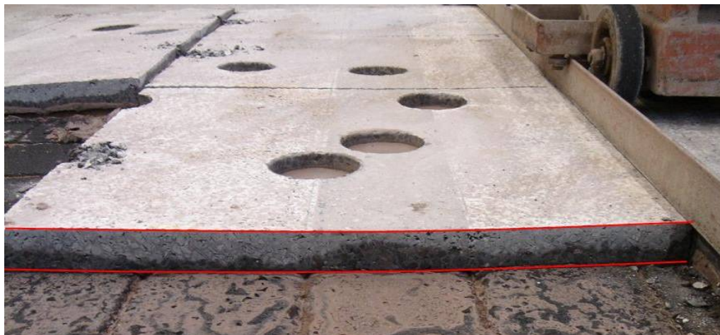
Figure 7.25 – Negligible deformation within the surface course
