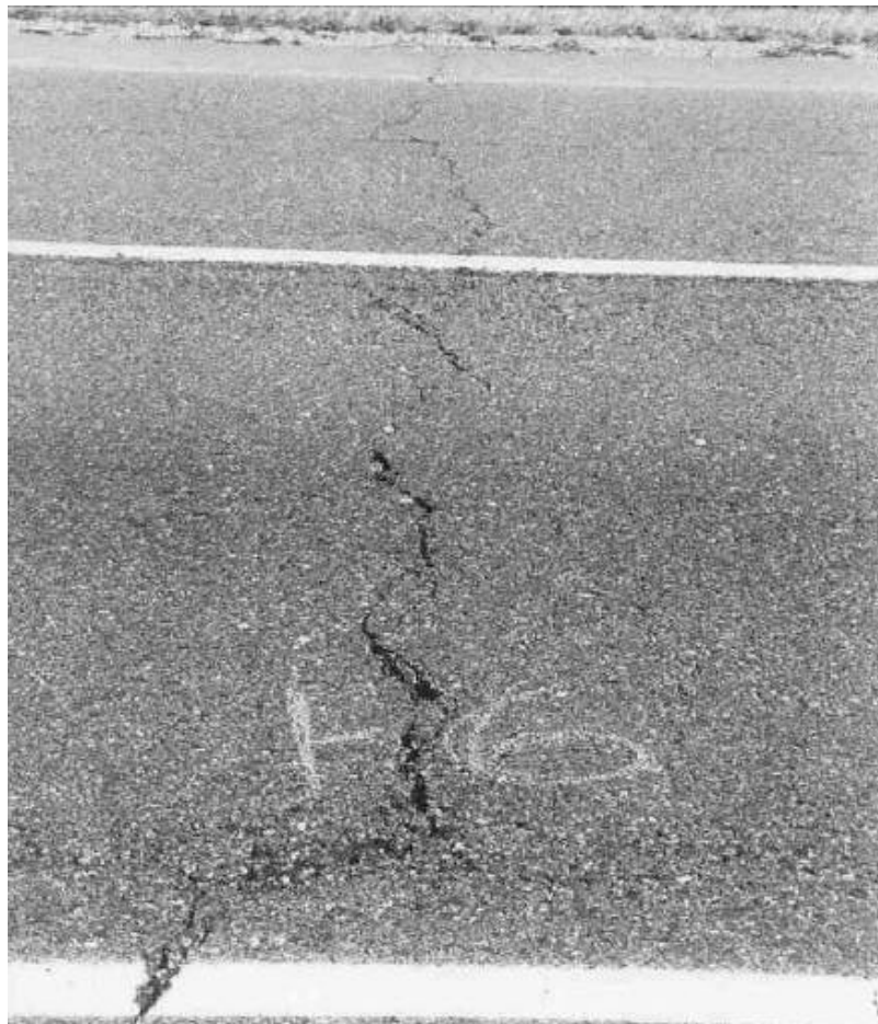
Figure 2.11 – Transverse reflective crack in a composite pavement with an unjointed concrete base (Saraf, 1998)
