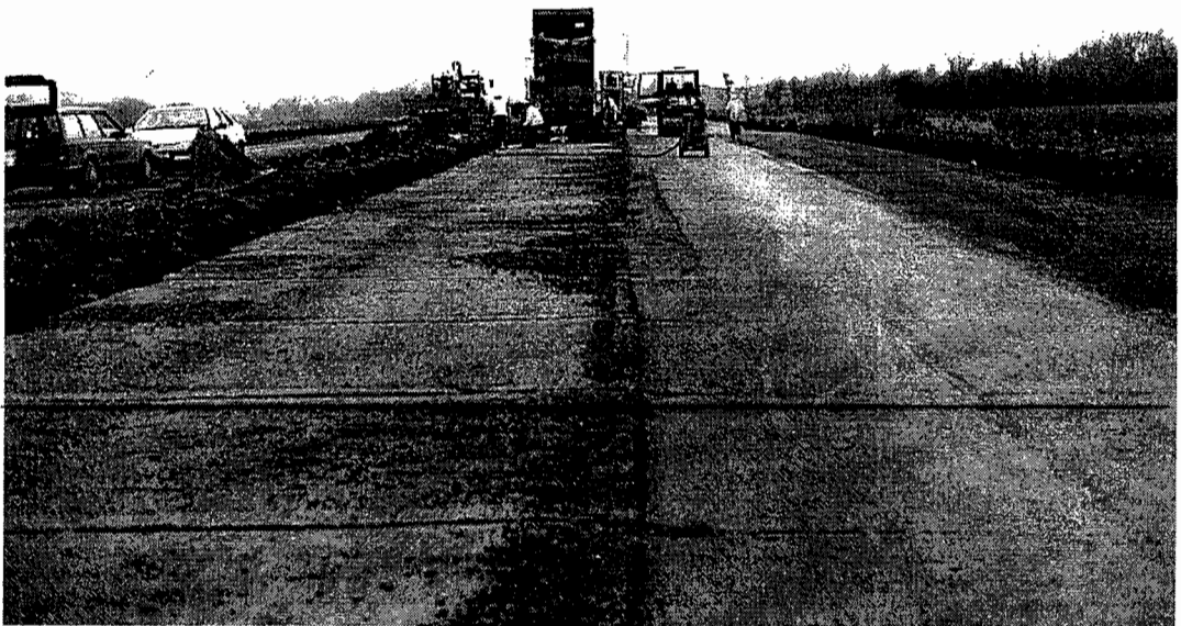
Figure 5.2. A slotted CBM layer before and after compaction
