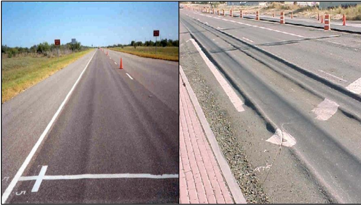
Figure 2.4: Different rutting severities in asphalt pavements (Soares 2005)
