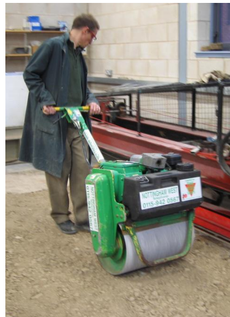
Figure 4. 12 Single drum vibrating roller used on Limestone for the PTF
