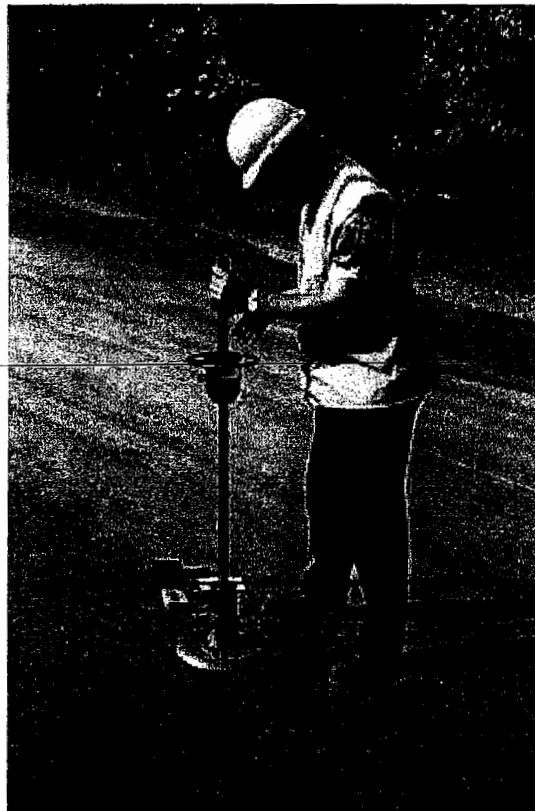
Plate 5-5 Dynamic Plate testing of the surface modulus of the sub-base
