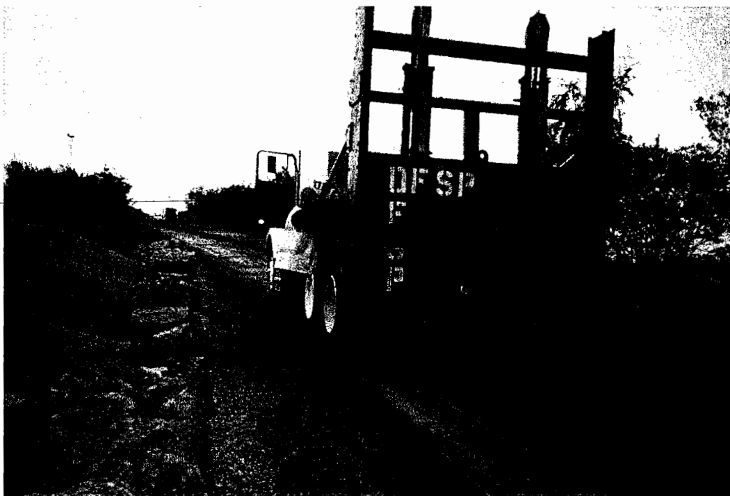
Plate 5-3 Guillotine breaker used to induce cracks in FRCBM
