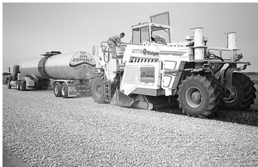
Figure 2-11 FDR reclaimer and stabilizing additive tanker (ARRA, 2001)
