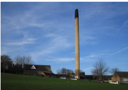
The chimney for the main boilerhouse at University Park
