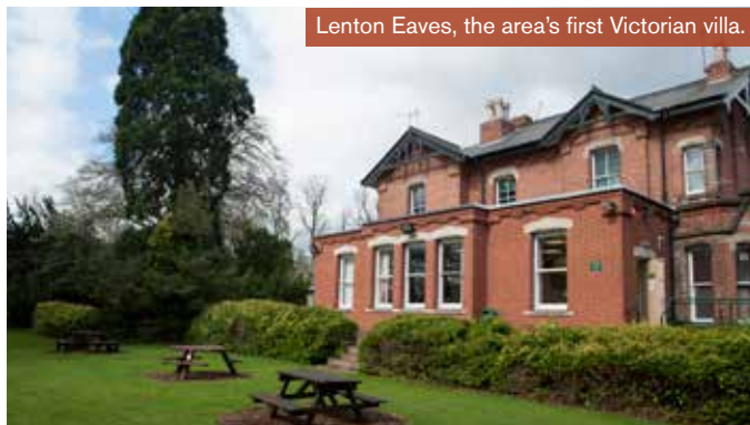
Lenton Eaves, the area's first Victorian villa.
