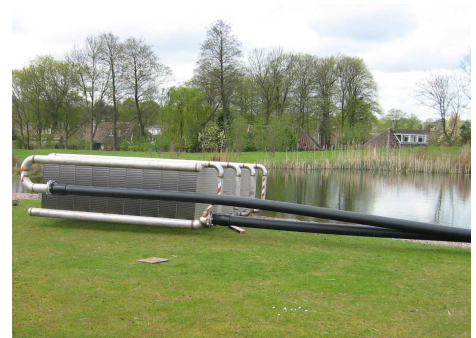
Heat pump system gets installed in the lake
