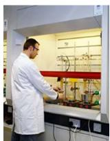
Fume cupboards are fitted in laboratories for the protection of users but, if not properly controlled, the fans can use large amounts of electricity and large volumes of heated or cooled air can be lost from the building. The Estate Office has been working with academic schools to raise awareness of the issue, liaising with technical managers, labelling fume cupboards and monitoring energy use.
